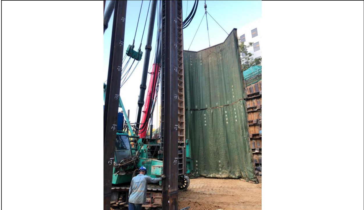
Hoisting of noise barrier during piling
