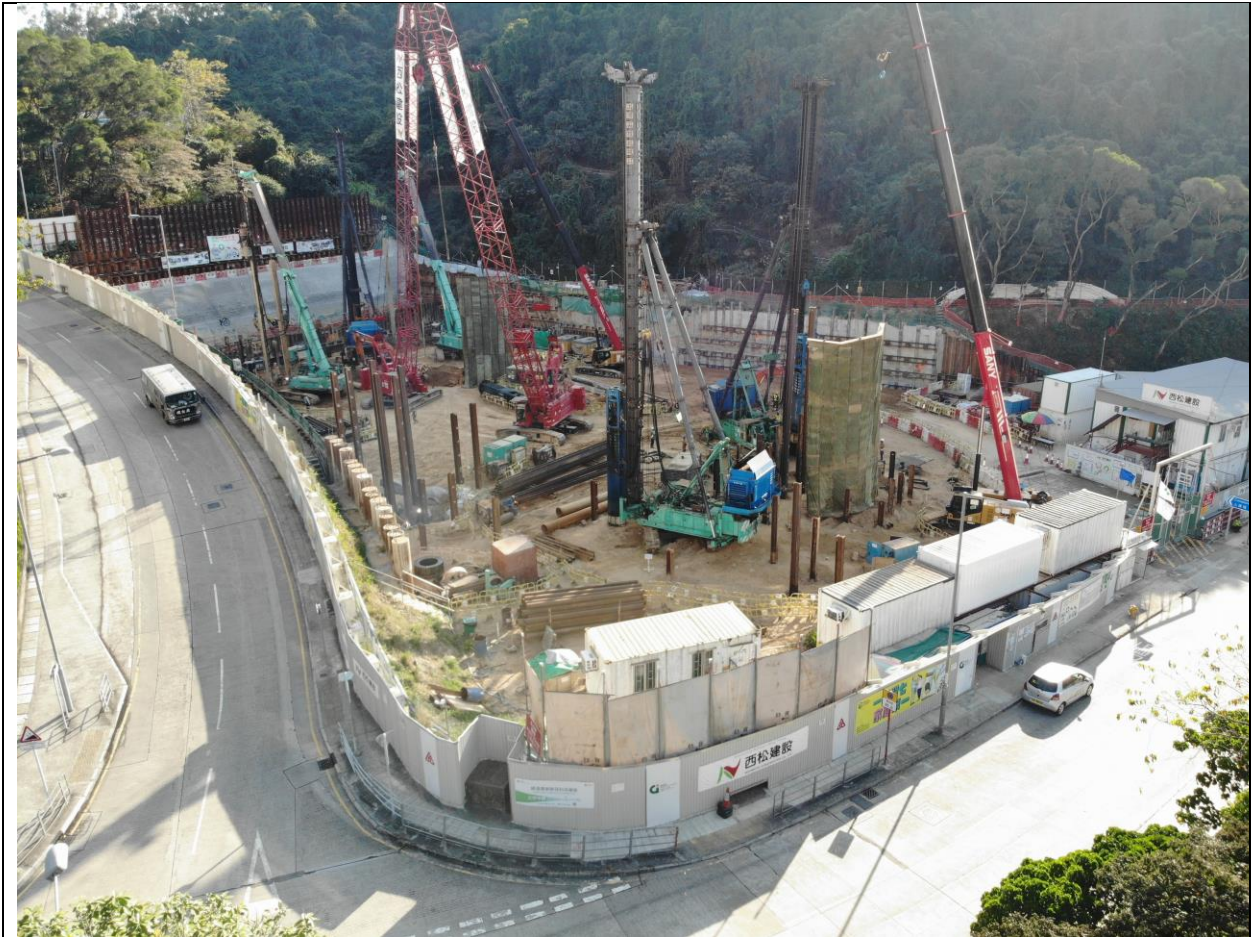
Hoisting of noise barrier during piling
